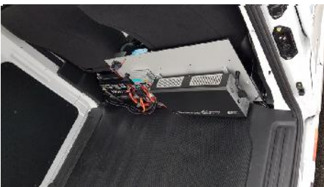
Inverter and Lilon Battery
